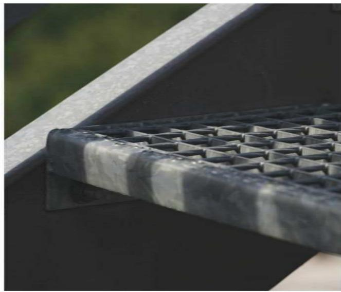
The treads can be easily and quickly mounted to the existing structure using four screws.
