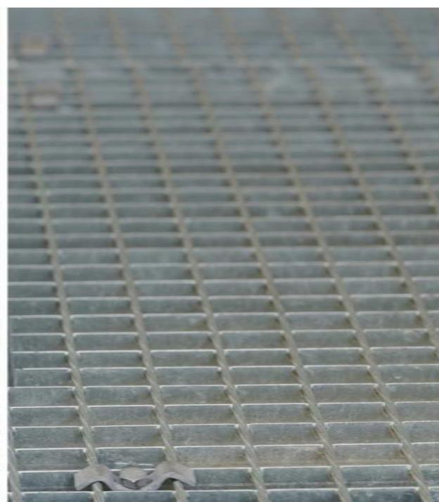
The elements forming the grating structure are load-bearing flat bars and twisted cross rods with a diameter of 5 mm or 6 mm (depending on the thickness of the load-bearing flat bar). **The load-bearing flat bars are responsible for transferring the loads acting on the grating, while the cross rods provide positioning and stability to the load-bearing flat bars.**
